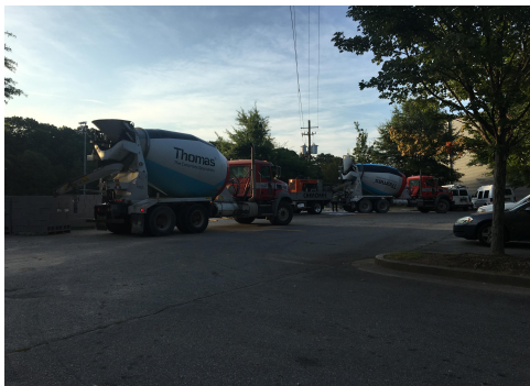
FD- 7AM Concrete Pour- 5 trucks to complete Slab on Grade
