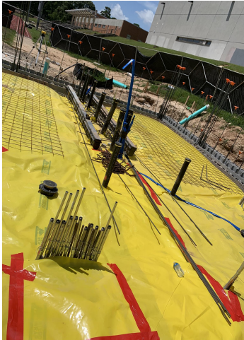
FD- Vapor Barrier Installation
