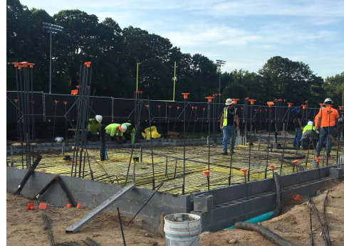
FD- Welded Wire Fabric and Slab on Grade Rebar Installation
