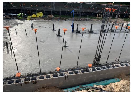
FD- Poured Slab on Grade- Prep for Troweling
